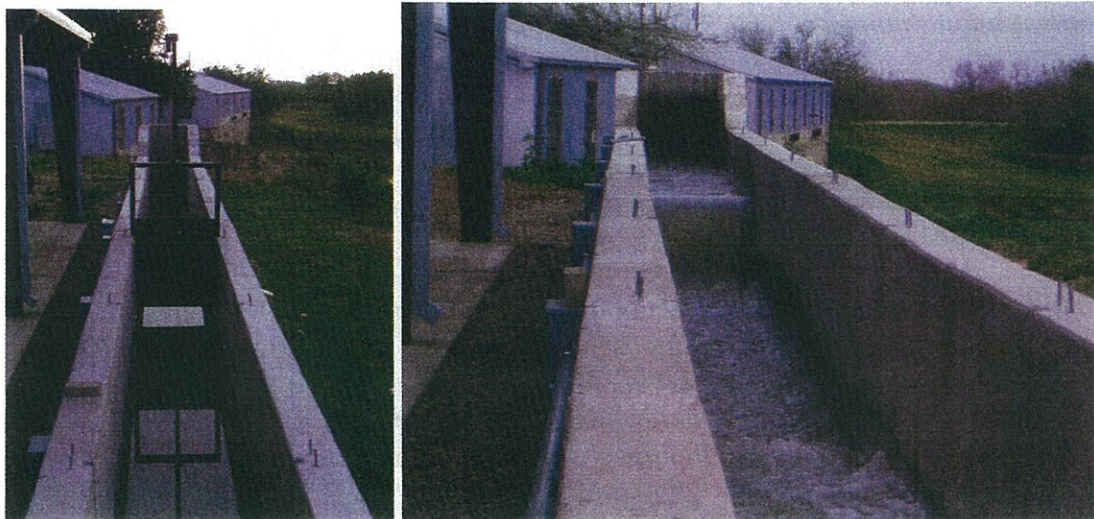
Figure 5: Automated flume gate and metering flume at the Harlingen Irrigation District training facility
