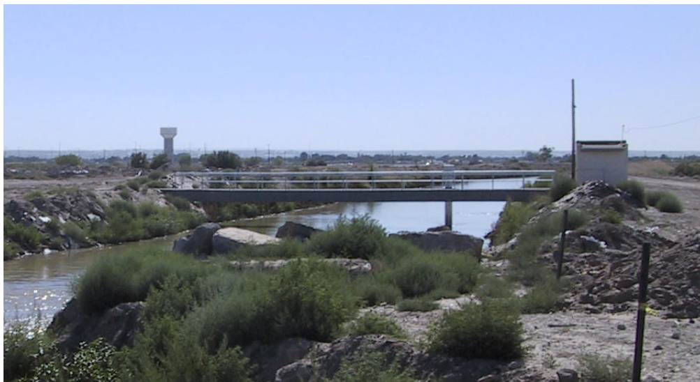
Figure 1 – Open Channel Meter Bridge
