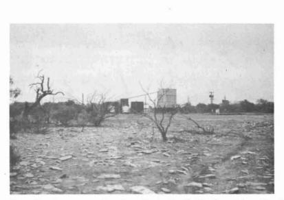
E. Waterflood system in the Burkett field, in John Sanders Survey 162, 11/2 miles north of Burkett. Note leveled surface pit in right background. Apparent overflow or discharge from previous pit has eroded surface soil (rock masses in foreground). Drainage is into tributary of Pecan Bayou. View is southeast.
