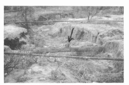
C. Previous method of salt water disposal into North Prong Hords Creek, in section IO, T&NO RR Co. Survey, 1/2 mile north of Glen Cove. Surface is sand of the Trinity Group. Note vent on large pipe indicated by arrow. View is east.
