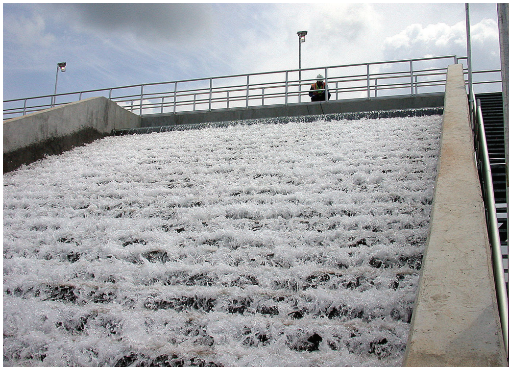
Figure 10-2. Cascade aeration, first step of treatment process.
