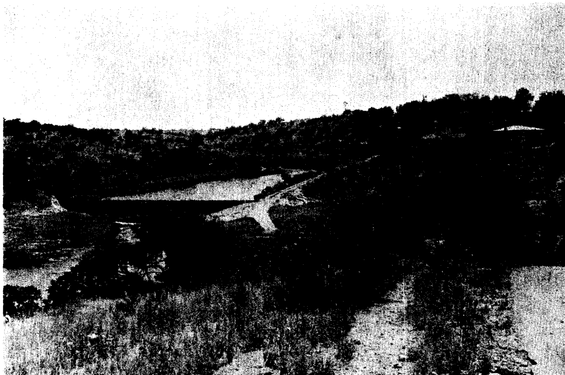
Figure 43.—Deep Creek Springs Reservoir
