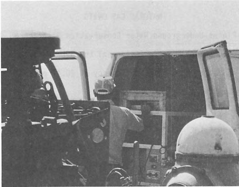
Dan Seale is checking the efficiency of a pumping plant.
