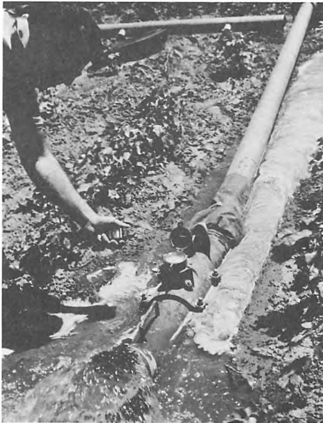
Ken Carver is metering water with a flow meter.
