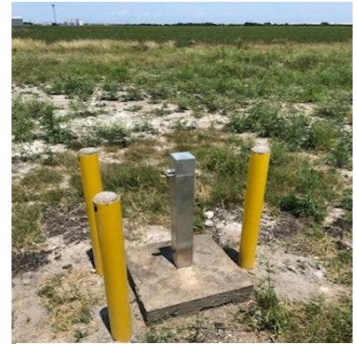
Monitoring Well at Site 1 (MW-1D)
