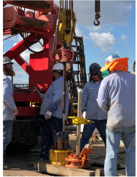
Installation of Monitoring Well at Site 1
