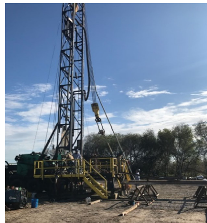
Drilling rig at Site 1 during Phase I
