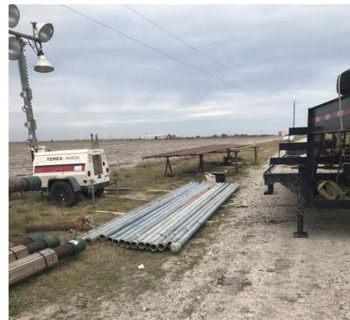
Temporary well casing
