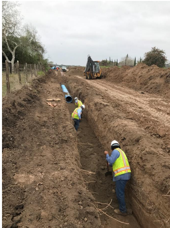
Figure 12 Photo, 12.15.16, District crews laying pipeline. Westward view.
