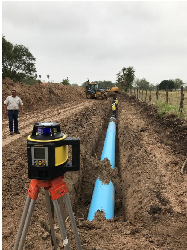
Figure 13 Photo, 12.15.16, District crews laying pipeline.
