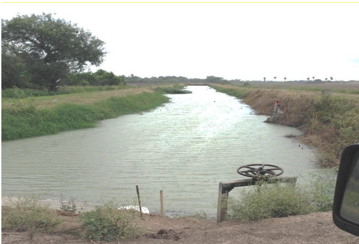
Figure 4 Saldaña Canal, Test Day.
