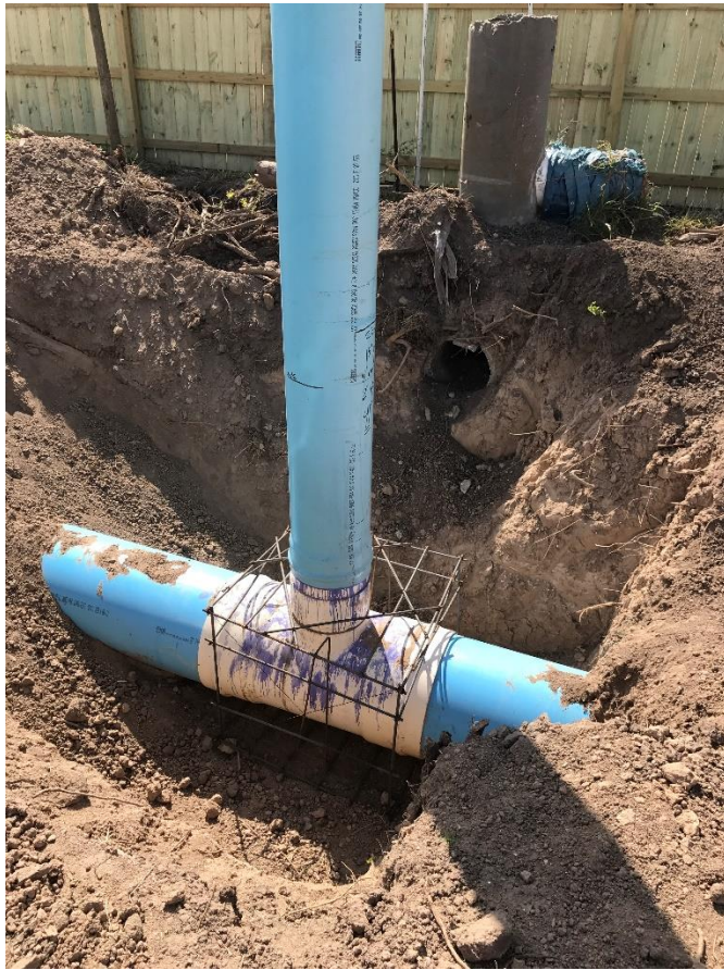
Figure 14 Photo, 2.17.17, rebar partially installed for saddle outlet.
