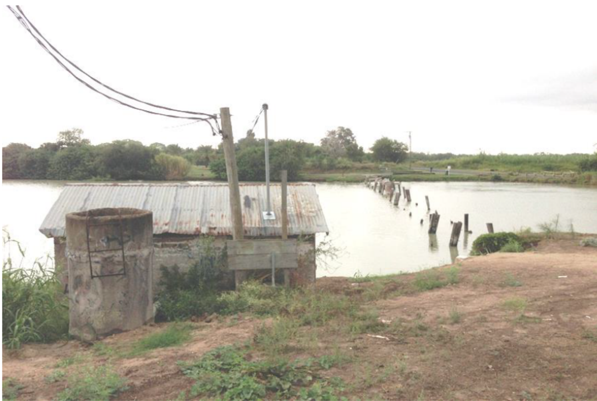
Figure 5 Saldaña Pump to be replaced in Phase II.
