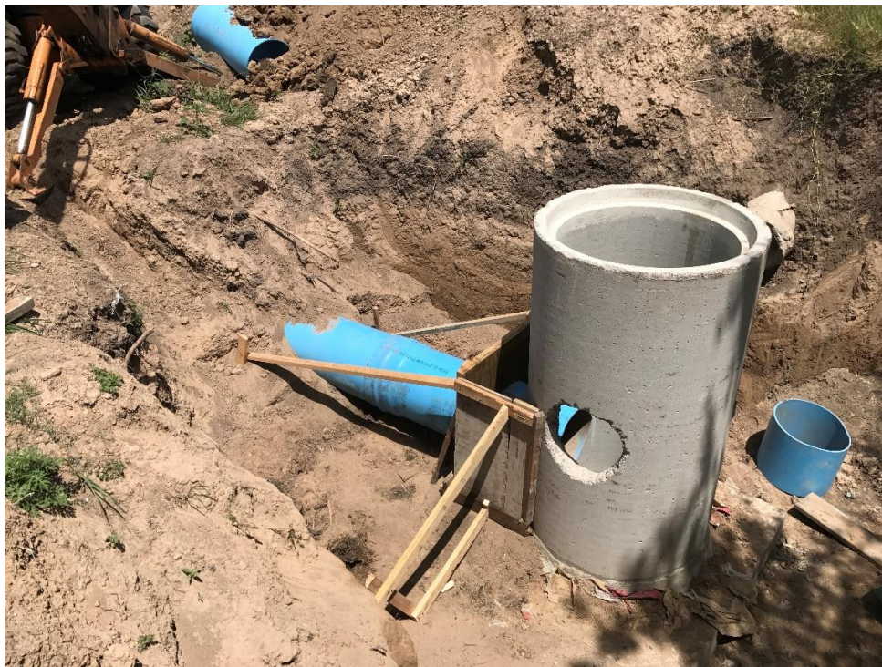
Figure 15 Photo, 4.20.17, pipes being connected to east end well.
