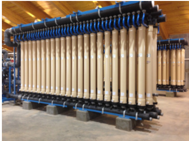
Microfilters at the Raw Water Production Facility Photo Credit: Eva Steinle-Darling
