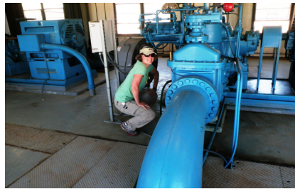
Sampling at Moss Creek Lake Pump Station
