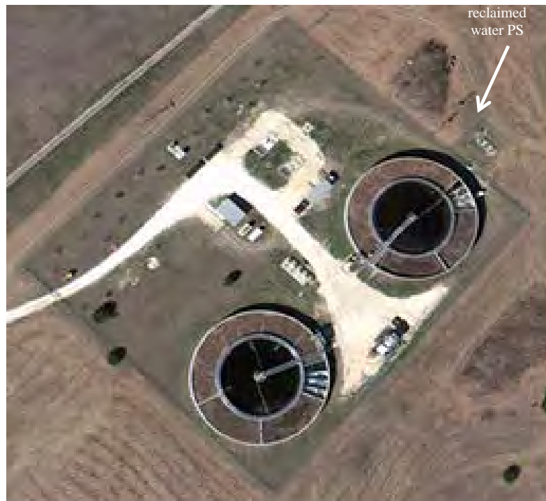
Figure 5-3: Kyle wastewater treatment plant.
