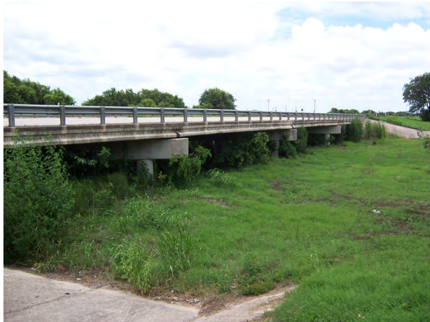
Figure 3.0 – Parkers Creek at Hwy 90 Eastbound
