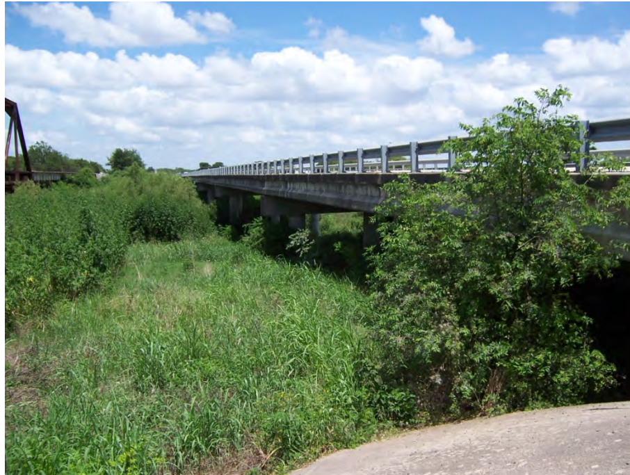
Figure 1.0 – Seco Creek at Hwy 90 Westbound
