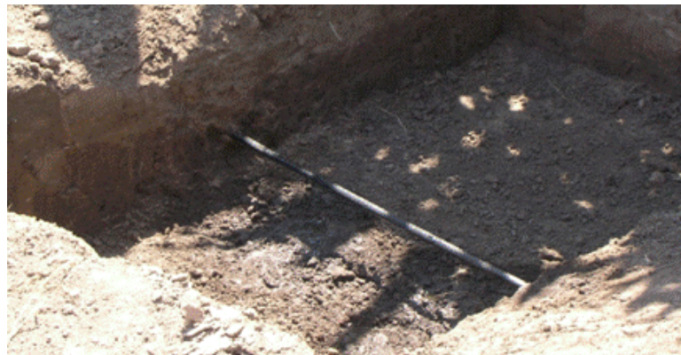
Figure 2.17. Excavation showing placement of Subsurface Drip Irrigation tape.
