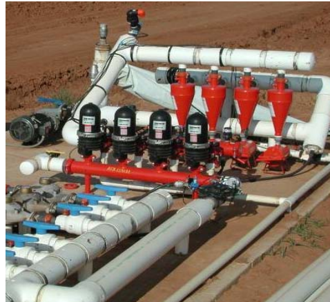
Figure 2.21. Sand media filters (left); hydrocyclone and disk filters (right) remove particulate matter from water to reduce risk of tape or emitter plugging.
