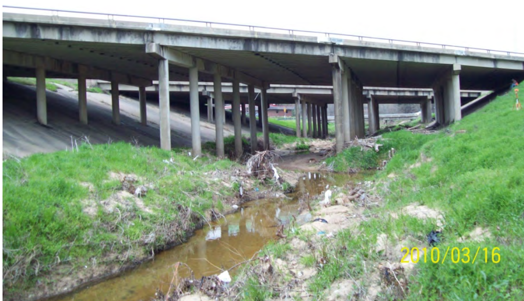
STR 08 downstream face
