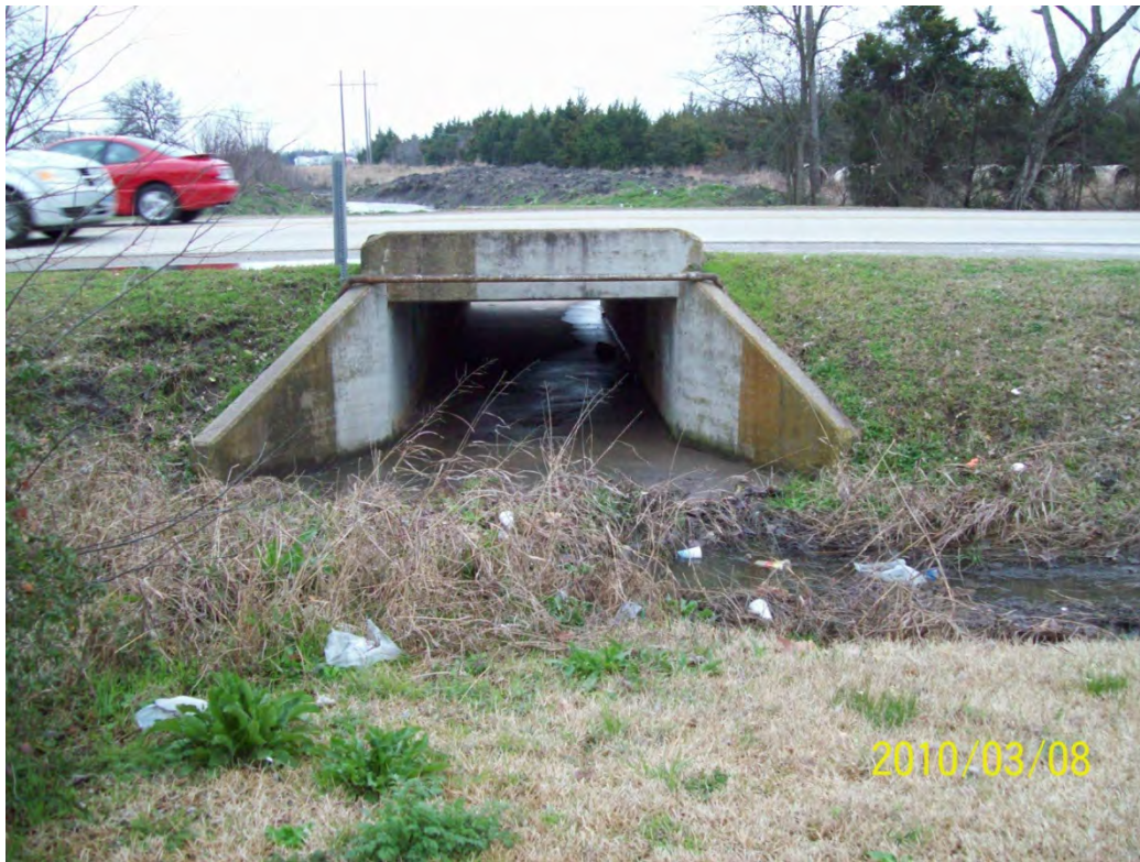
STR 02 upstream face
