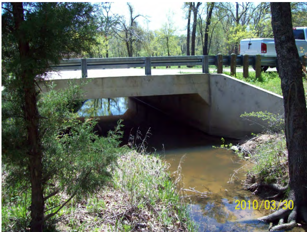
STR 19 upstream face
