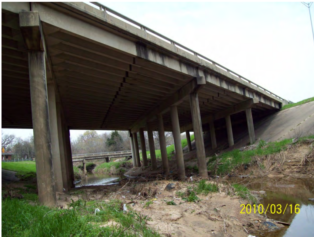
STR 07 downstream face
