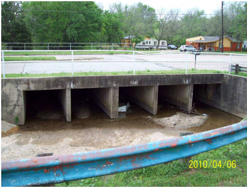
STR 21 upstream face
