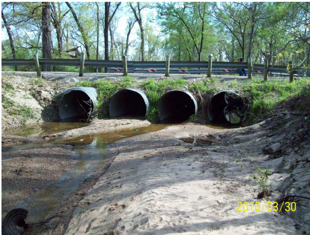
STR 22 downstream face
