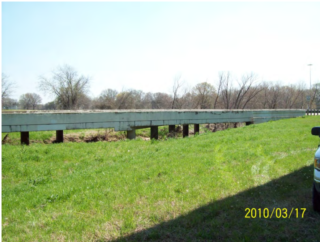
STR 11 – upstream face
