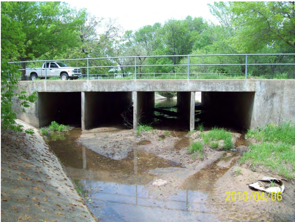
STR 25 downstream face
