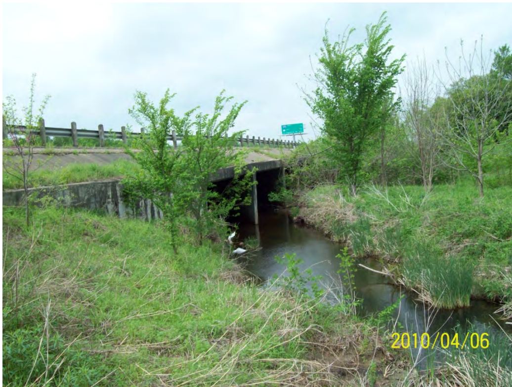
STR 24 upstream face
