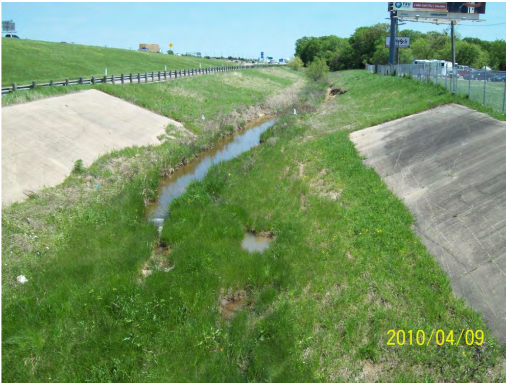
STR 33 looking upstream
