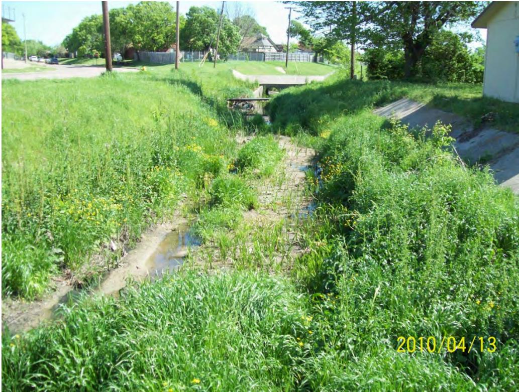
STR 27 looking upstream
