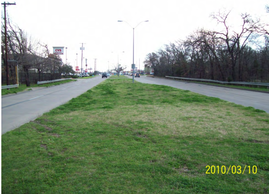
STR 05 looking east
