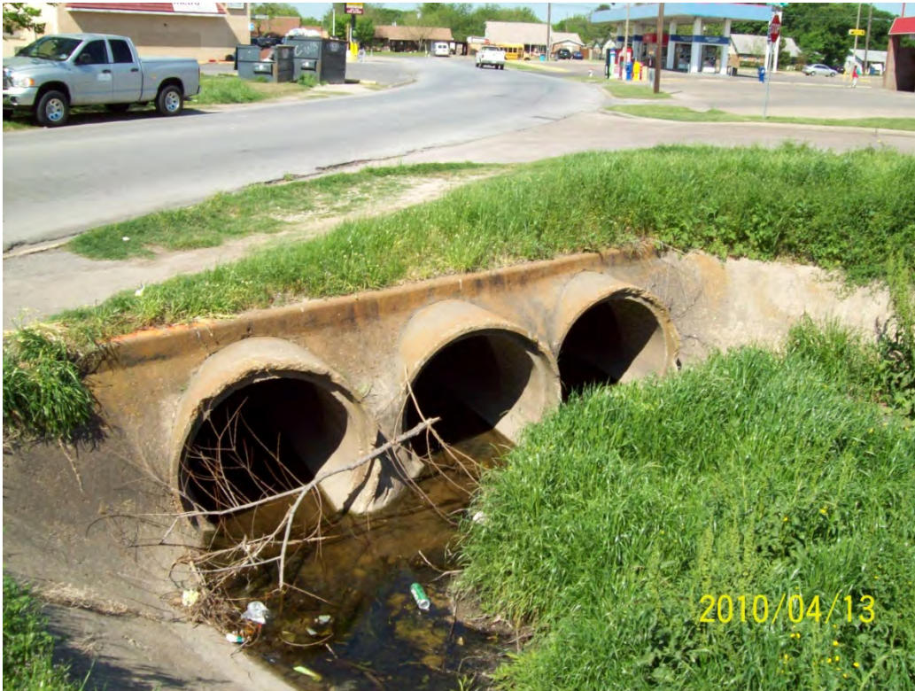
STR 27 upstream face
