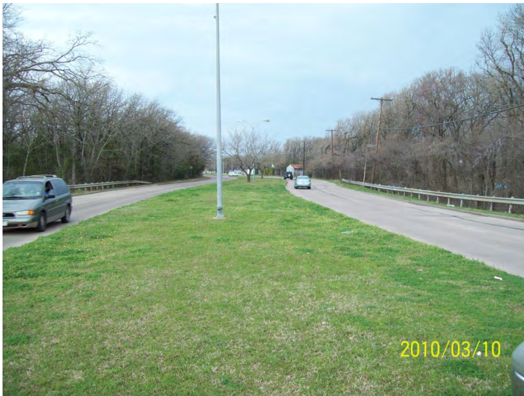
STR 05 looking west
