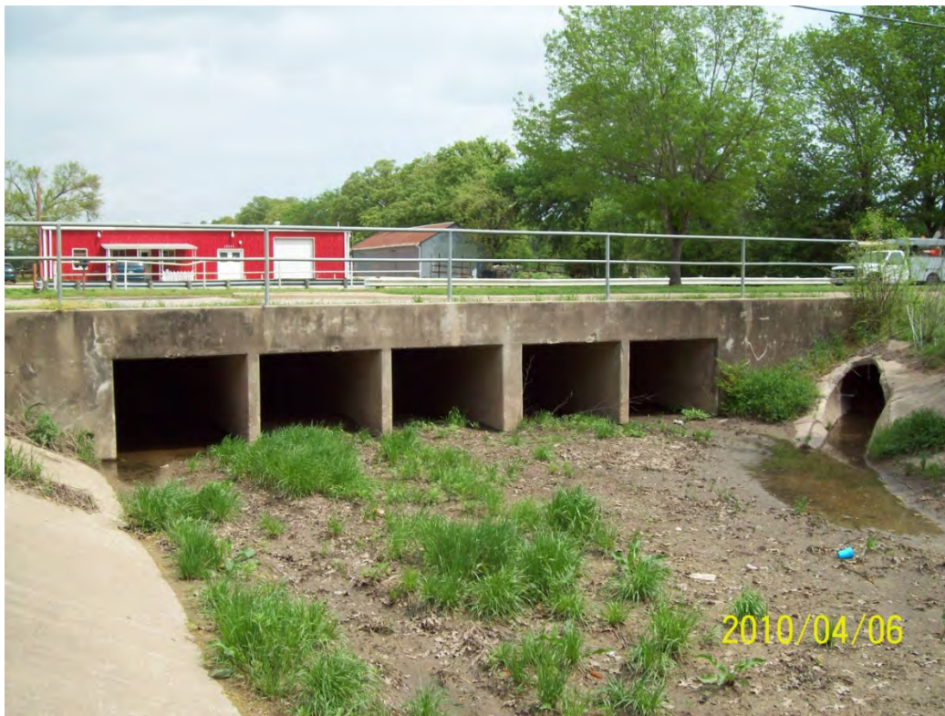
STR 21 downstream face
