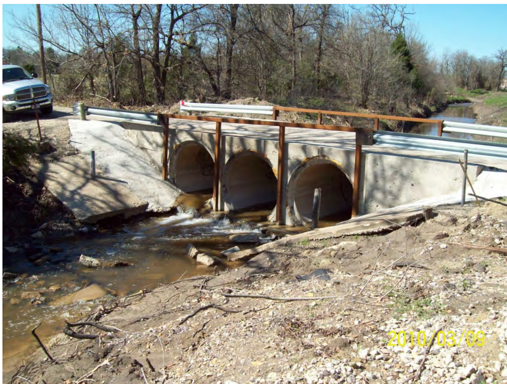
STR 04 downstream face
