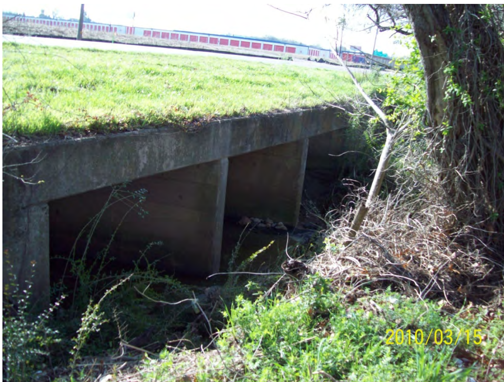
STR 18 downstream face
