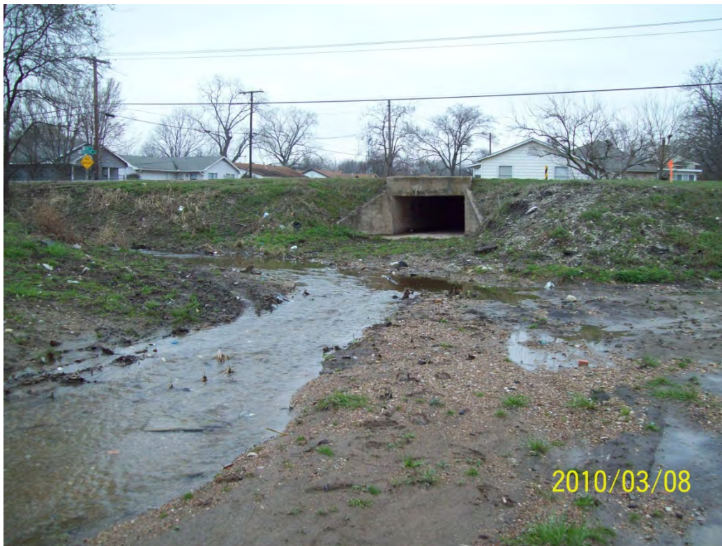
STR 02 downstream face
