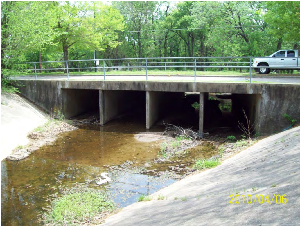
STR 25 upstream face
