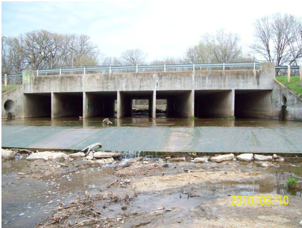
STR 05 downstream face
