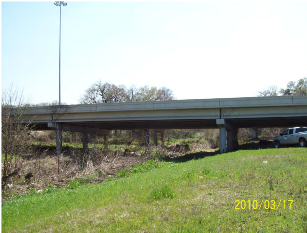
STR13 – upstream face
