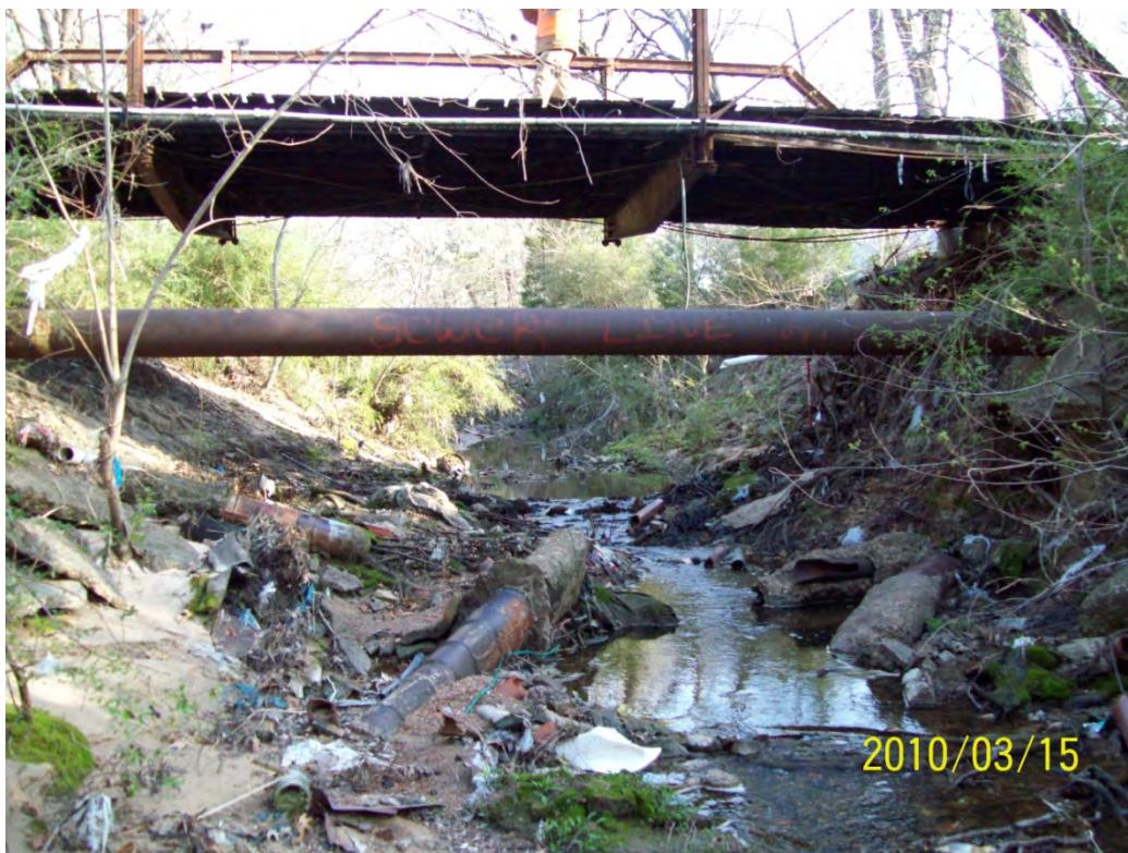
STR 06 downstream face
