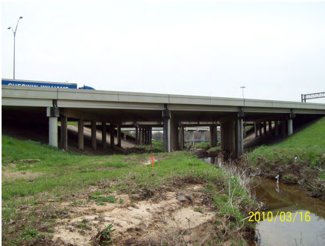
STR 07 upstream face
