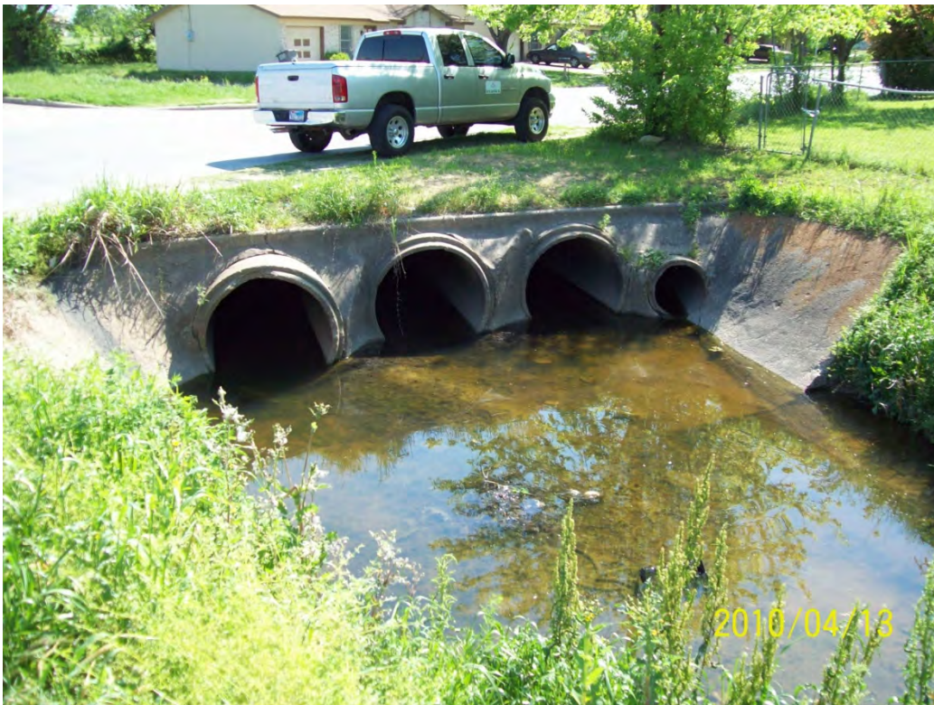
STR 27 downstream face
