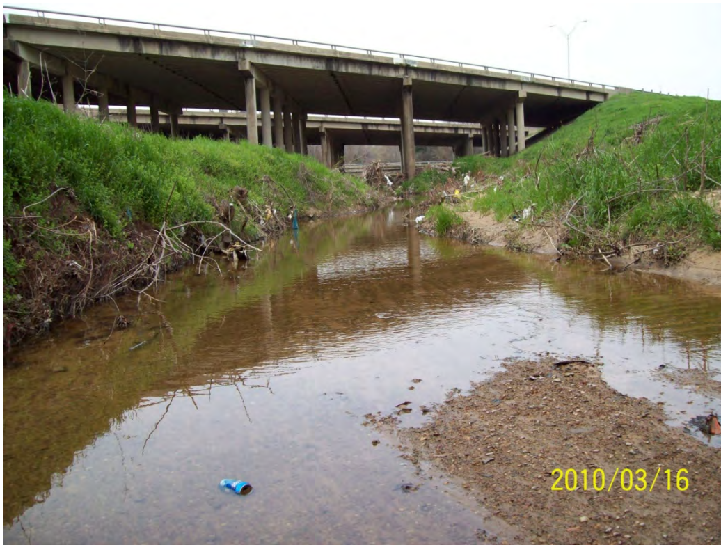
STR 09 – upstream face
