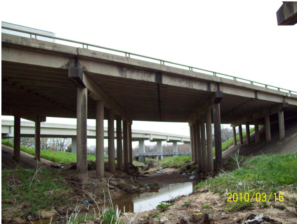
STR 08 upstream face
