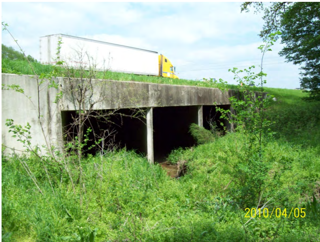
STR 20 downstream face
