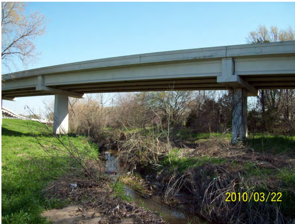
STR12 – downstream face
