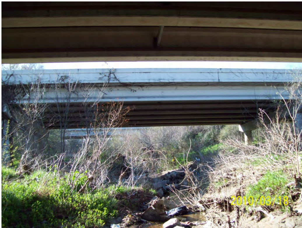
STR14 – upstream face
