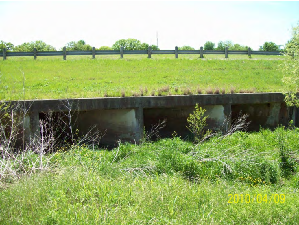
STR 32 downstream face
