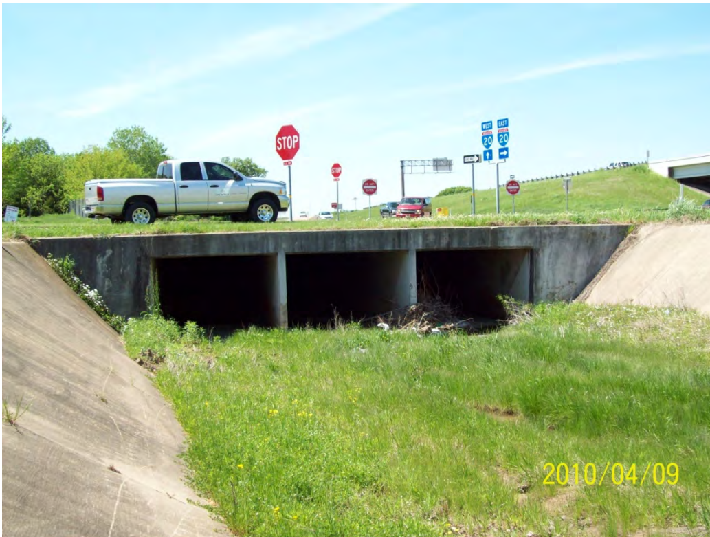
STR 33 upstream face
