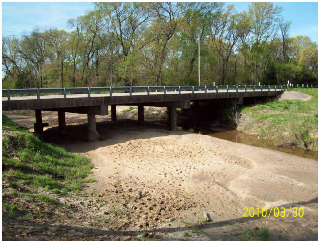
STR 16 upstream face
