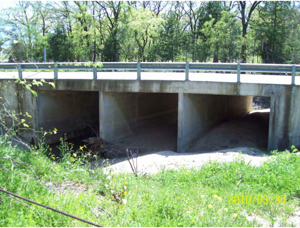
STR 23 upstream face
