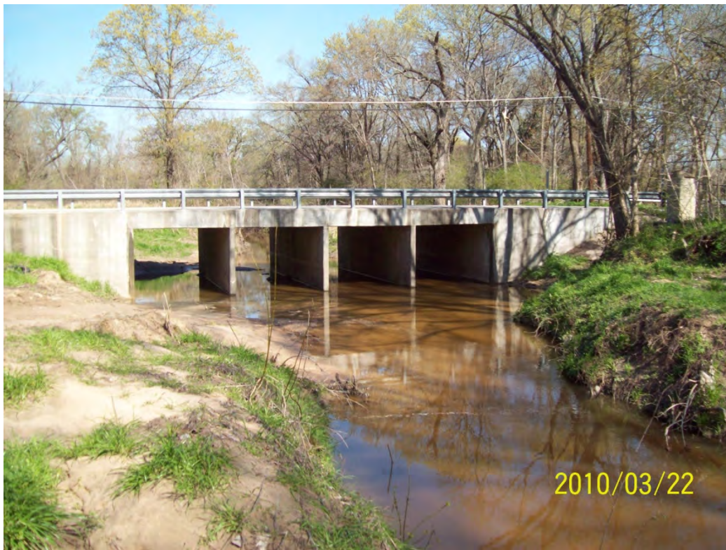
STR 17 – downstream face
