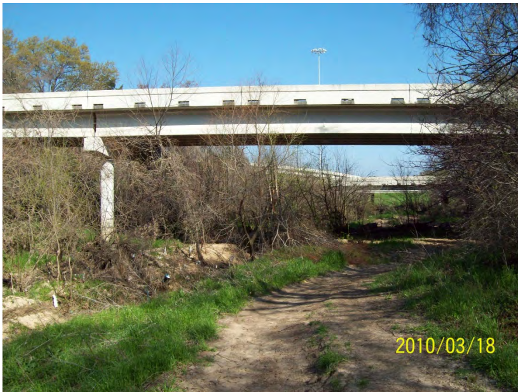
STR15 – downstream face
