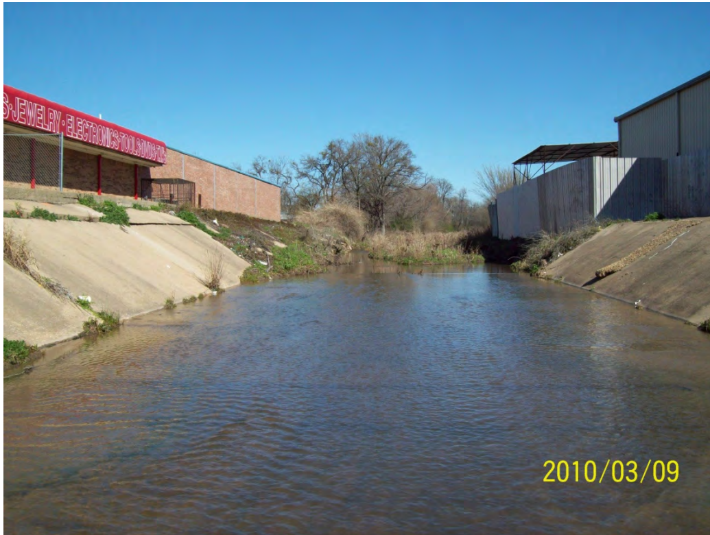
STR 03 looking upstream
