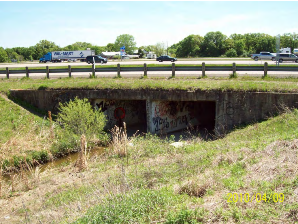
STR 35 upstream face
