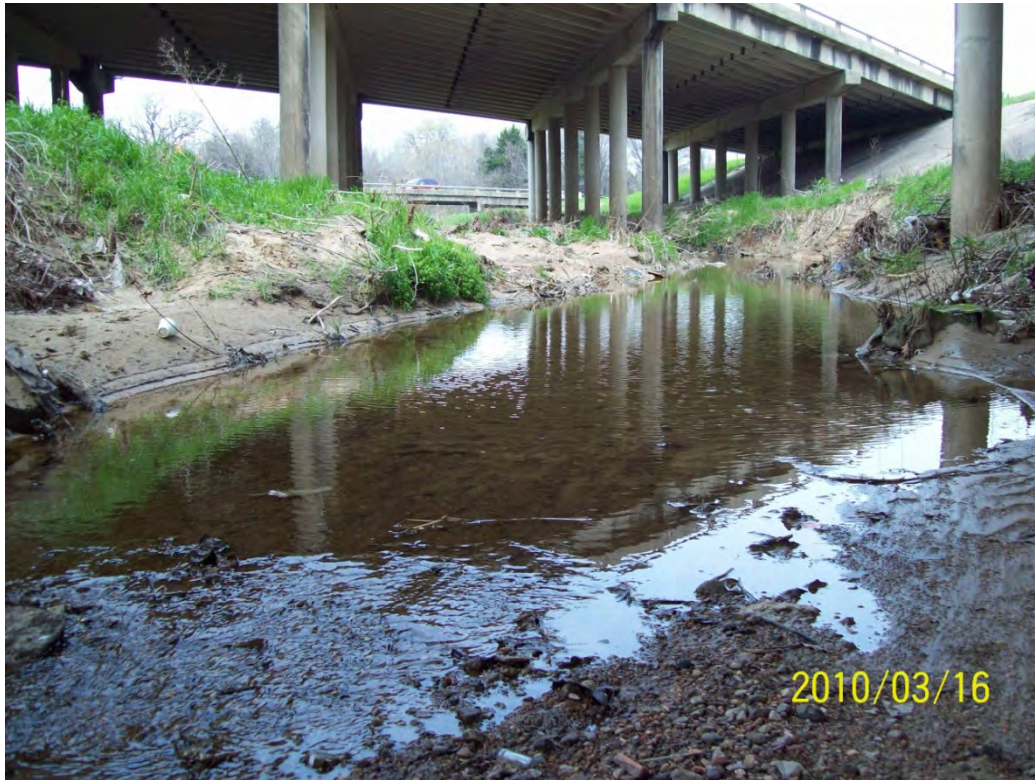
STR 08 looking upstream
