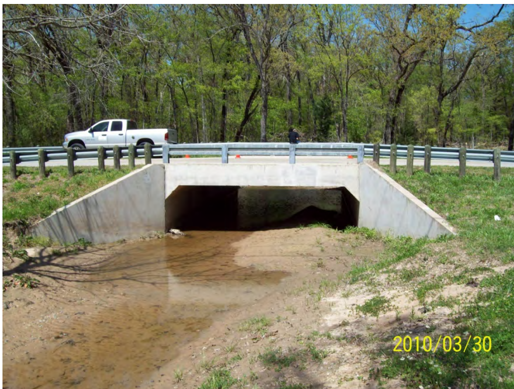
STR 19 downstream face
