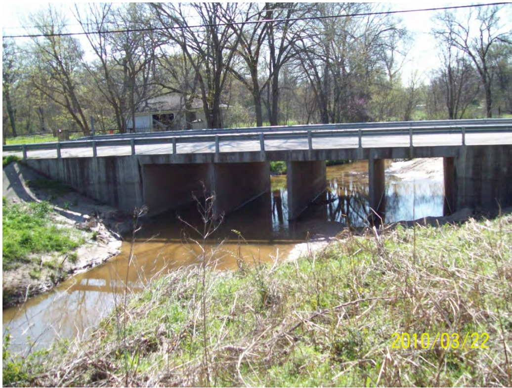
STR 17 – upstream face
