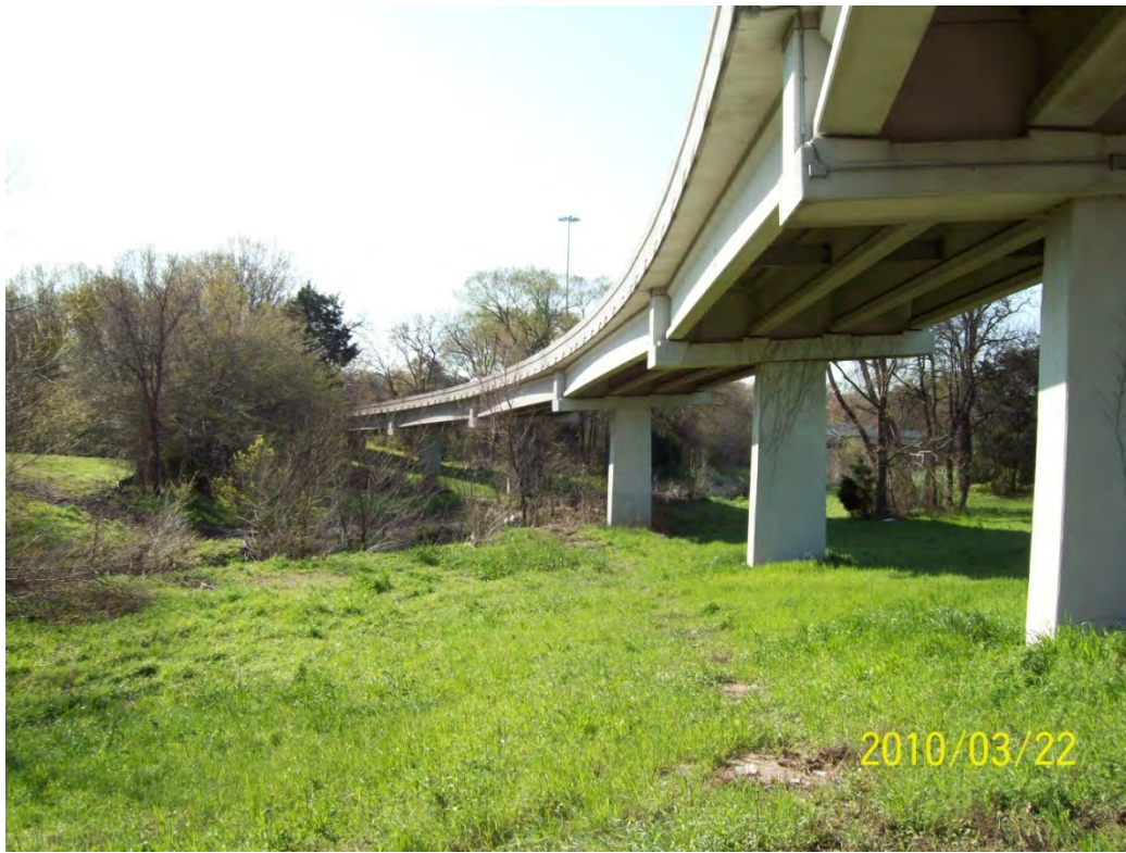
STR12 – upstream face
