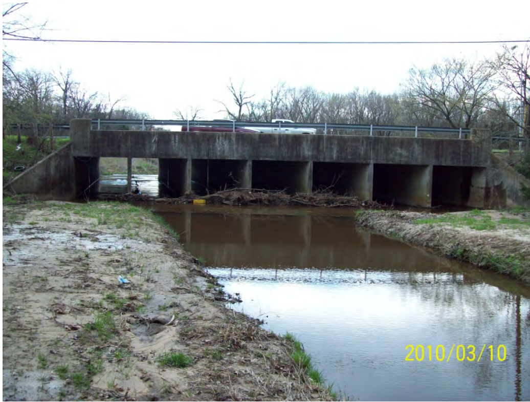
STR 05 upstream face
