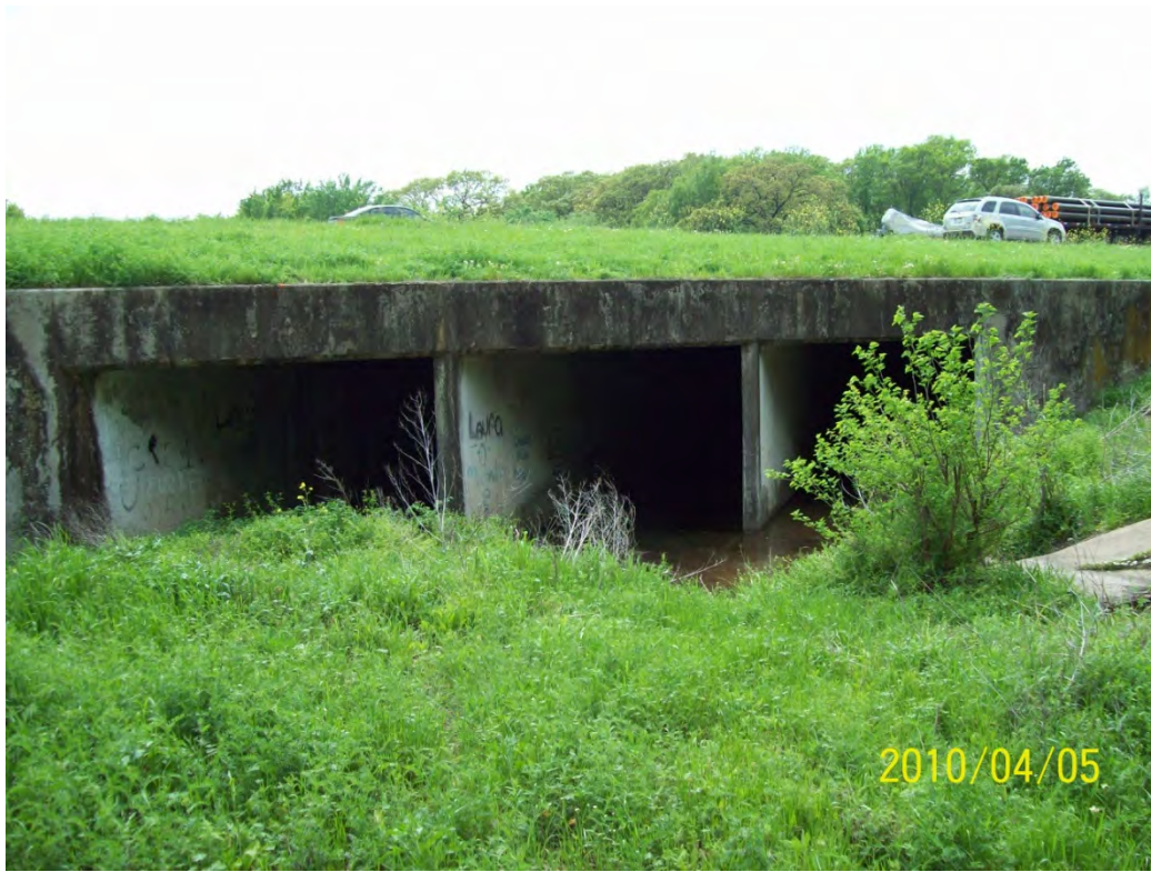
STR 20 downstream face
