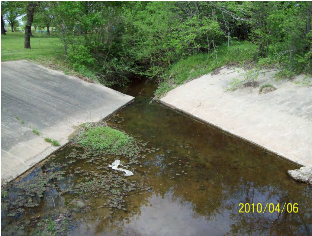
STR 25 looking upstream
