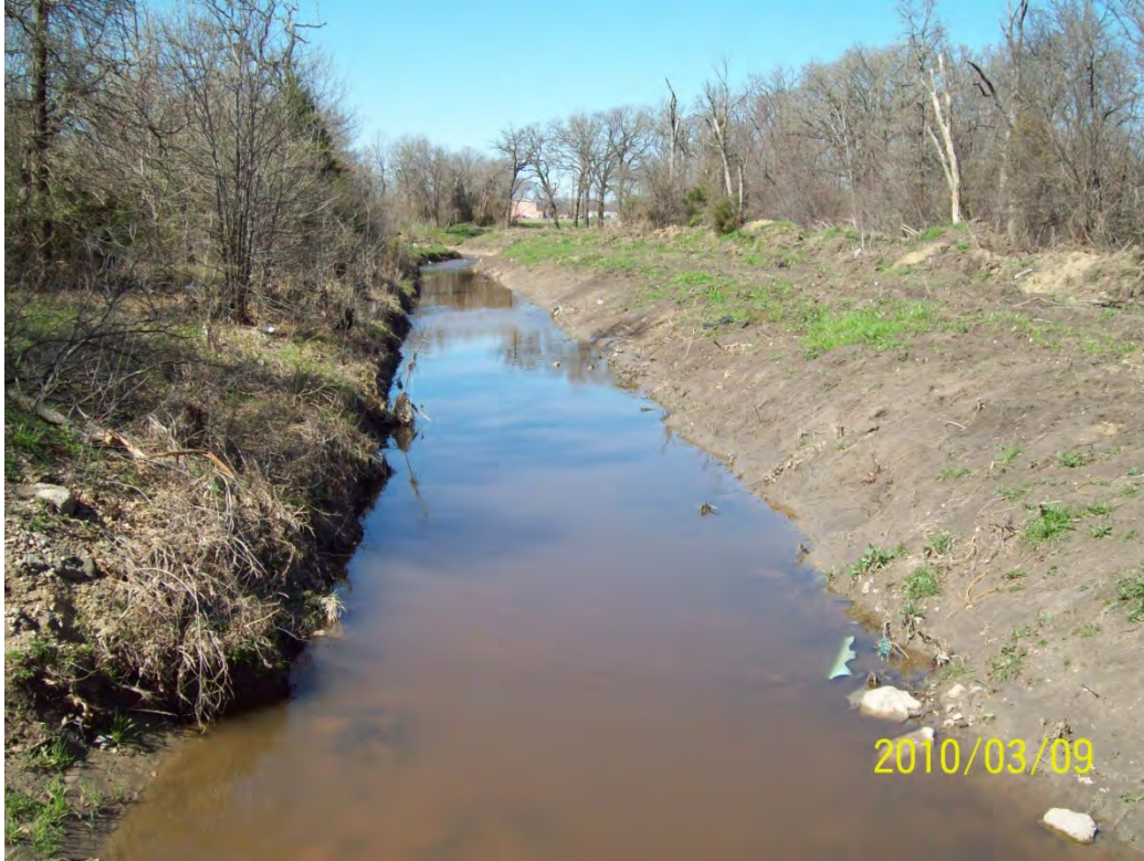
STR 04 looking upstream
