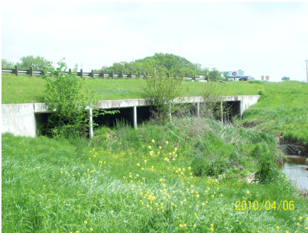
STR 24 downstream face
