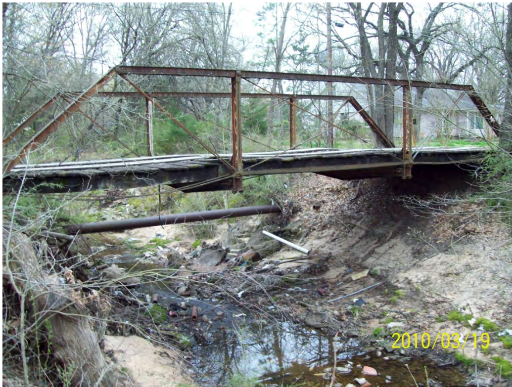
STR 06 upstream face
