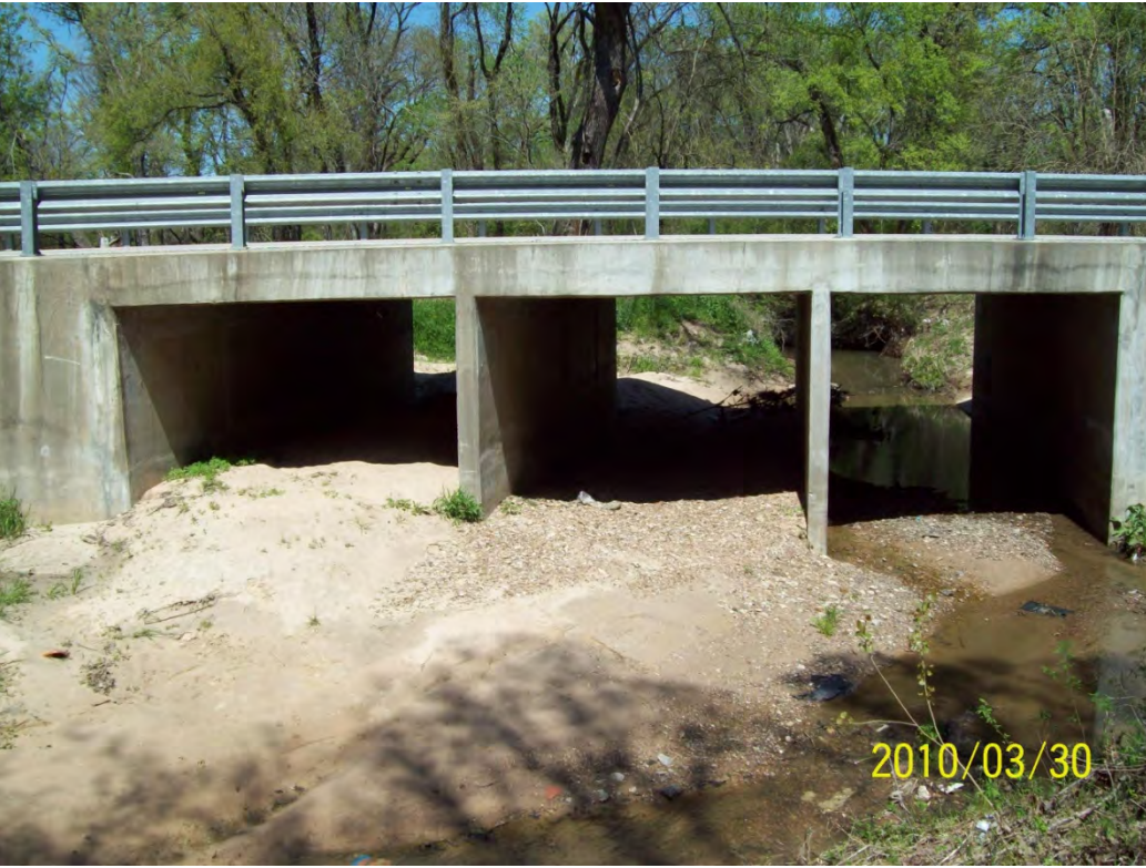
STR 23 downstream face
