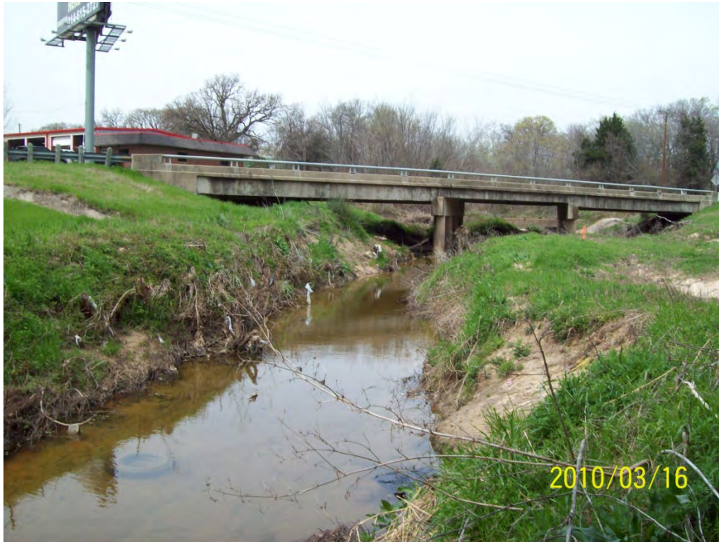
STR 07 looking upstream
