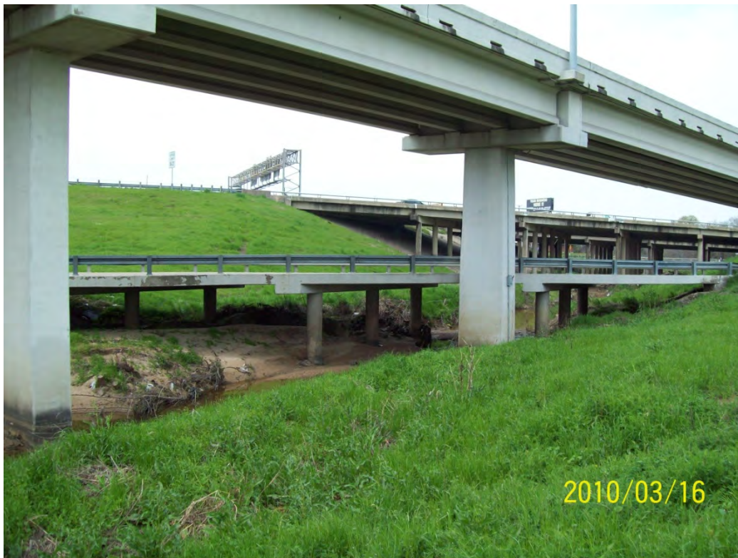
STR 09 – downstream face
