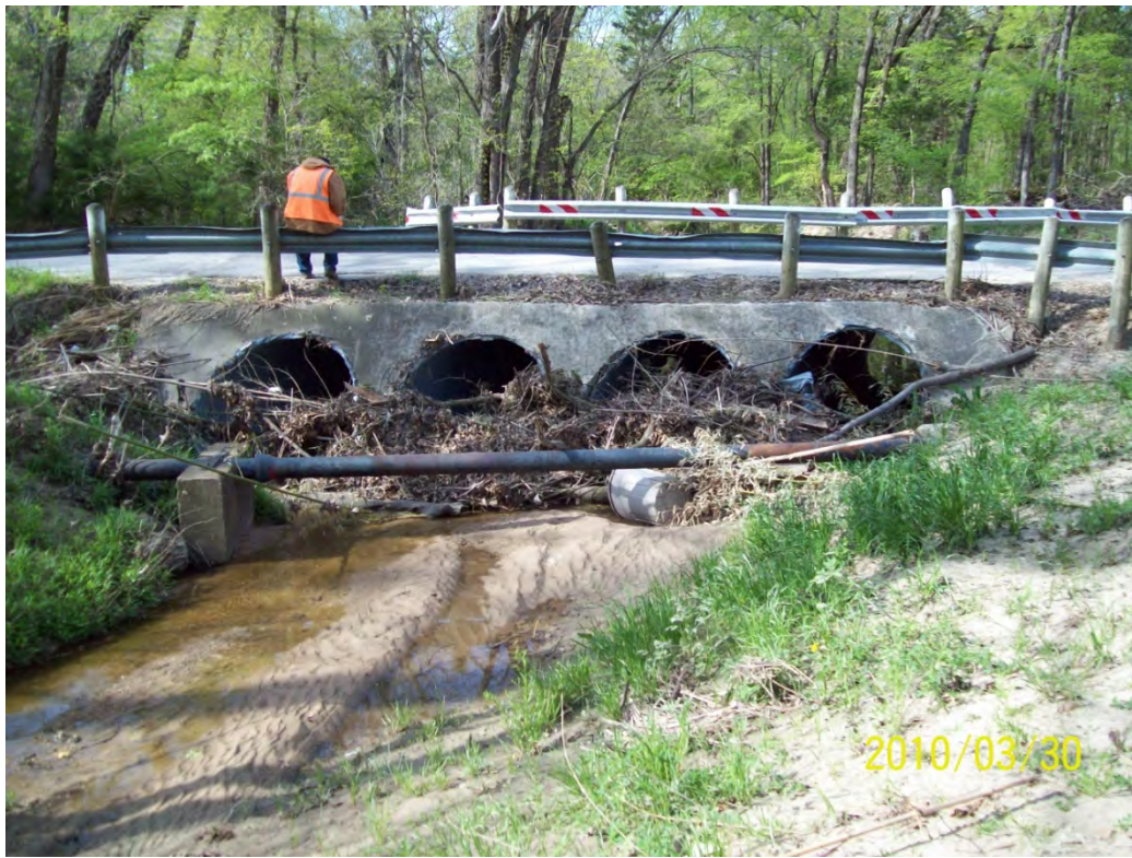
STR 22 upstream face
