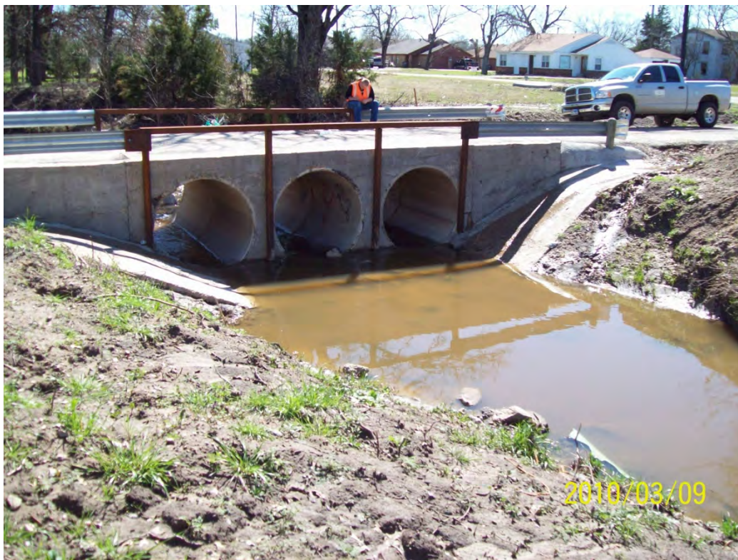
STR 04 upstream face
