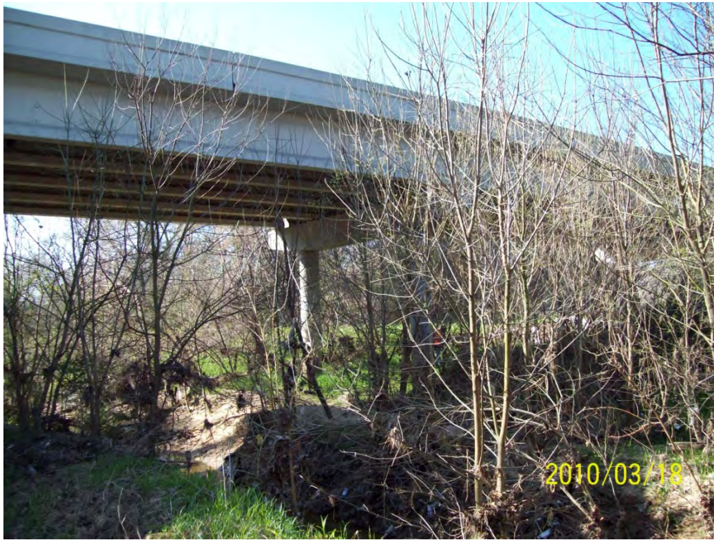
STR15 – upstream face
