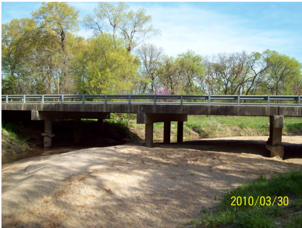
STR 16 downstream face
