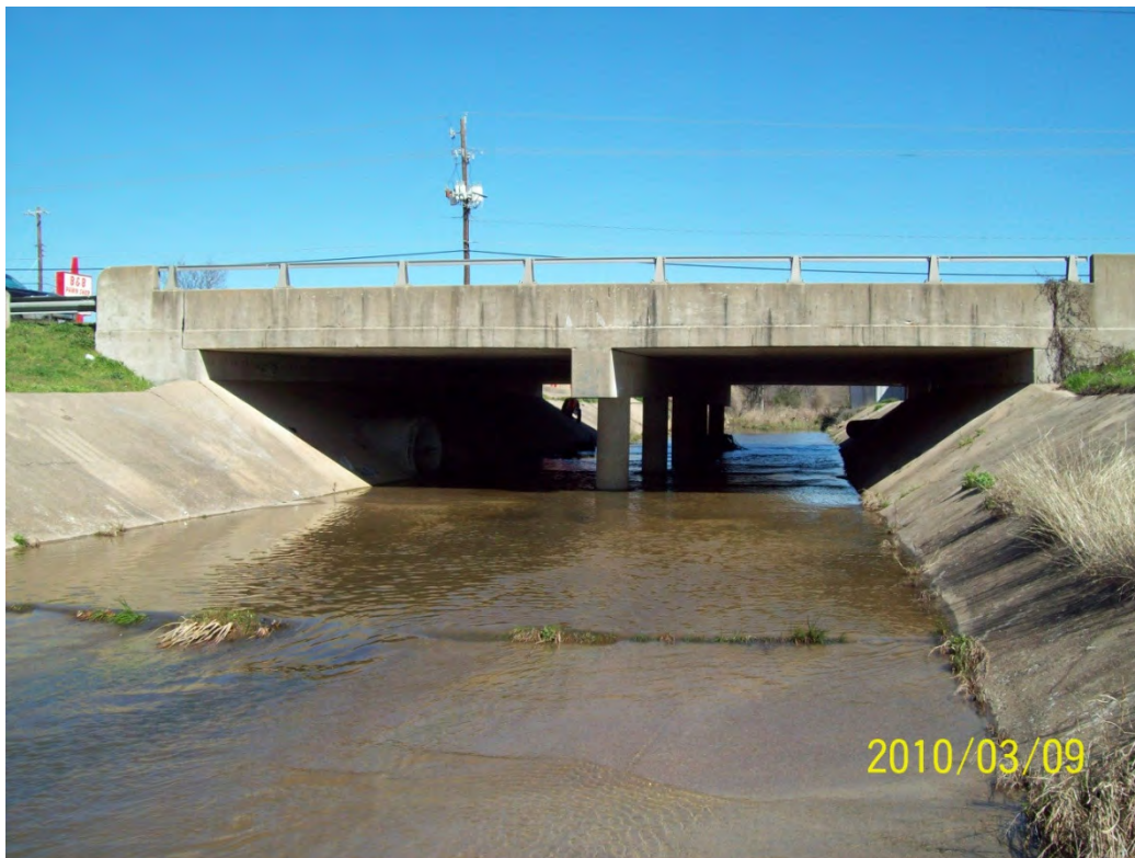
STR 03 downstream face
