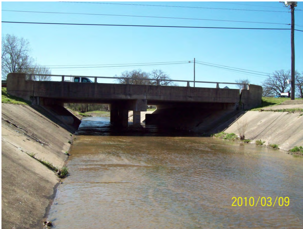
STR 03 upstream face
