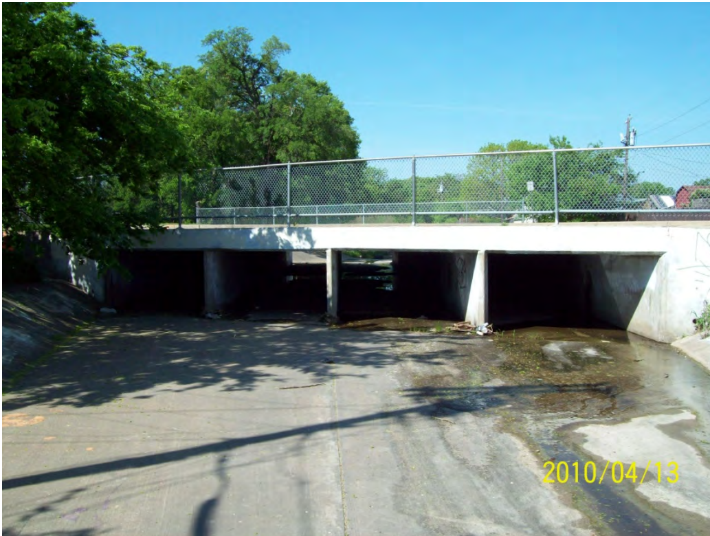
STR 26 upstream face
