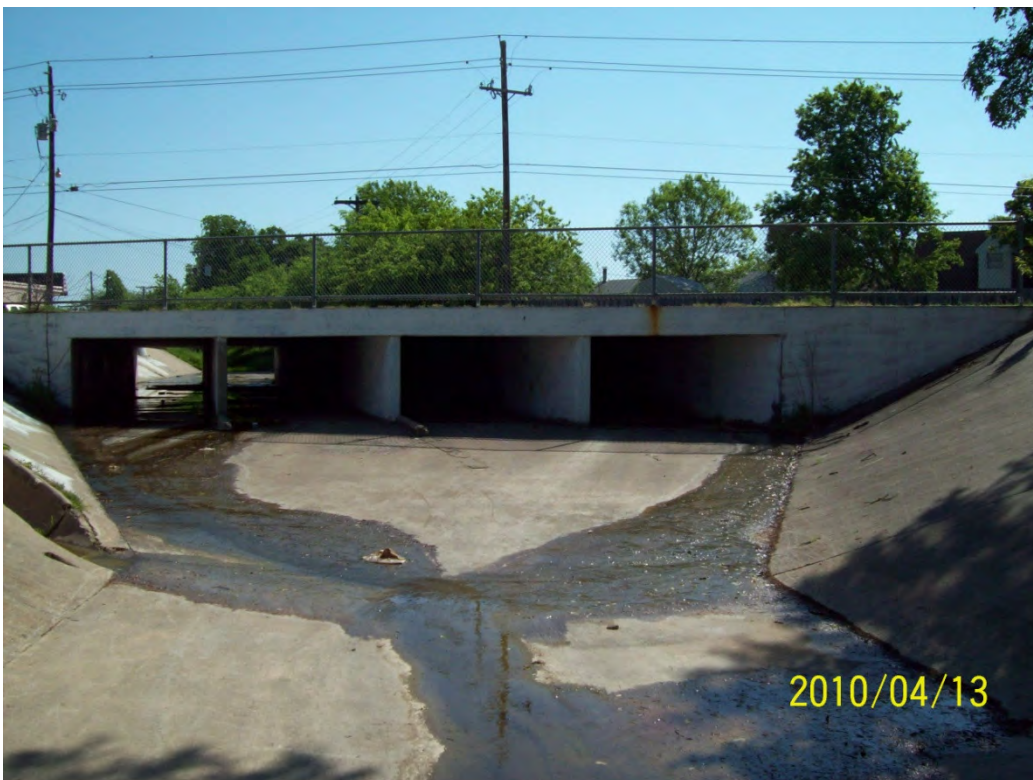
STR 26 downstream face
