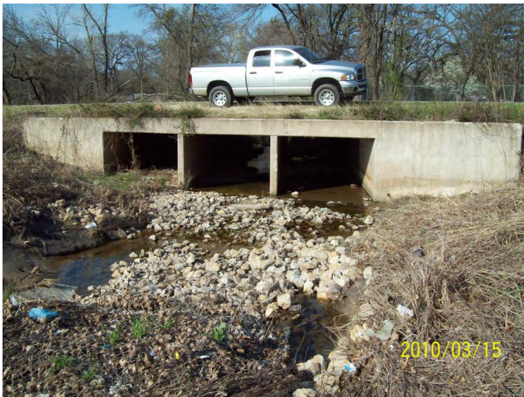
STR 18 upstream face
