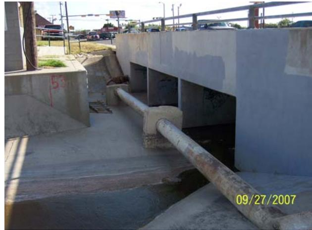
**Figure 7. Wastewater Line Crossing and Wall Obstruction Upstream of McPherson Avenue**
