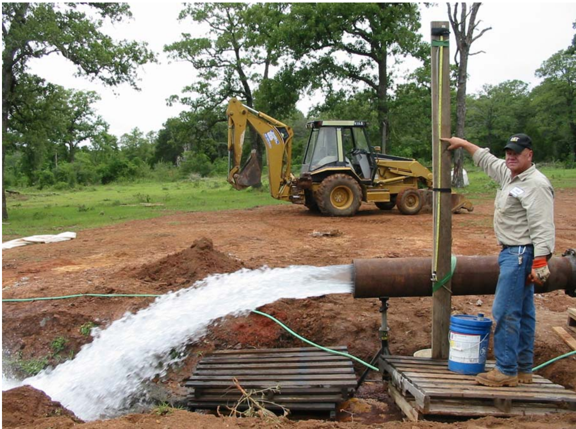
Figure 12 Pumping Test in Operation
