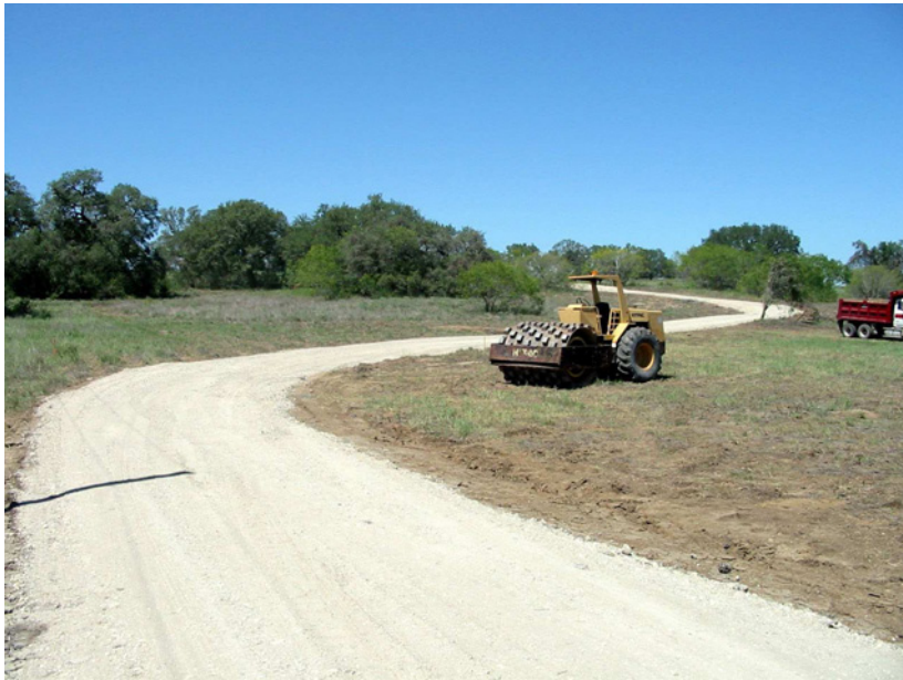
← a. ROAD PREPARATION
