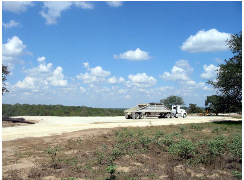
b. DRILL-SITE PAD CONSTRUCTION →
