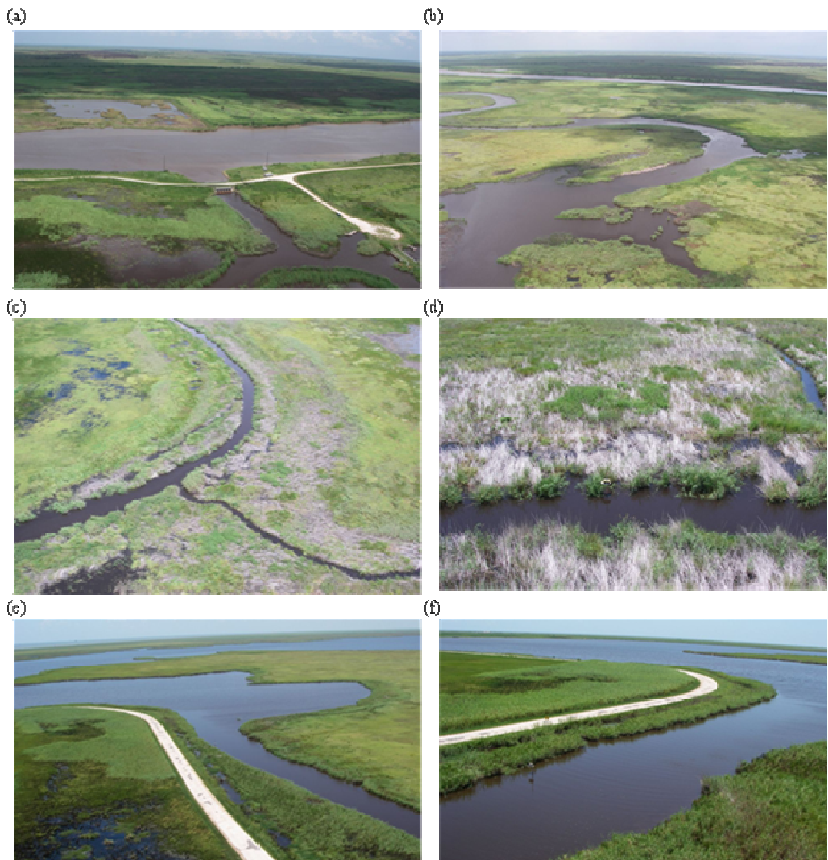
Figure 2.3 a) Star Lake Control Structure on the GIWW, b) Upper Five-mile Cut with GIWW in background, c) Five-mile cut, d) MCF2 station on Five-mile cut, e) Clam Lake juncture with upstream entrance to Ten-Mile Cut, f) MCF1 at upper Ten-Mile Cut, Clam Lake in background and downstream is to the left.
