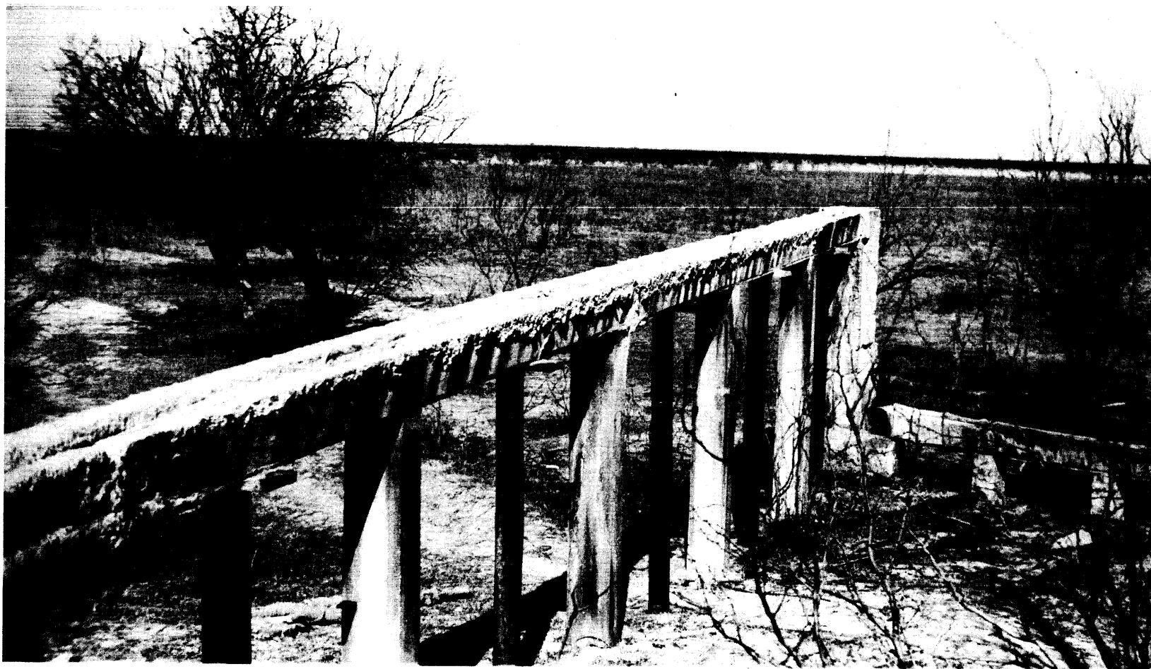
VIEW OF WELL BB-2 AND FLUME ABOUT 10 MILES SOUTHWEST ON BRACKETTVILLE, SHOWING DEPOSITS CONTAINING SULFUR ON FLUME
