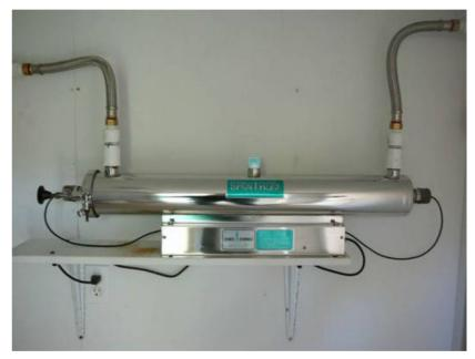
Ultraviolet filters for potable water system.
