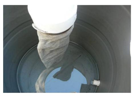
Sock filter to remove coarse debris.
