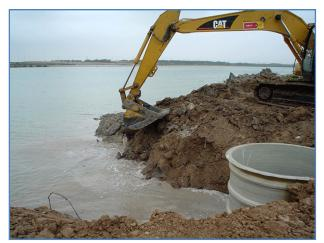
Figure 5 - Pilot plant stilling well intake on the Brownsville Ship Channel (north bank)
