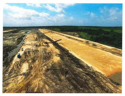
Figure 1 - Western Edge of Reservoir Placing Filter Sand
