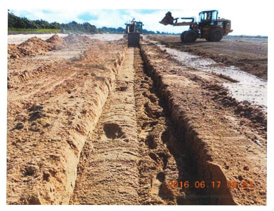
Figure 4 - Test Placement of Chimney Drain
