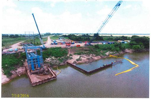
Figure 3 - Riverside View of Temporary Coffer Dam for River Outfall
