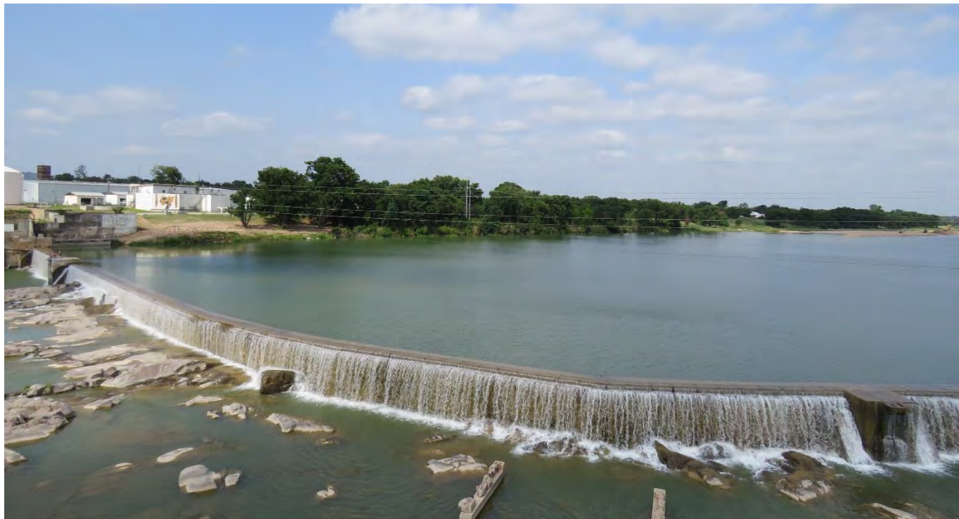
Source: Llano River Dam, Llano, TX
