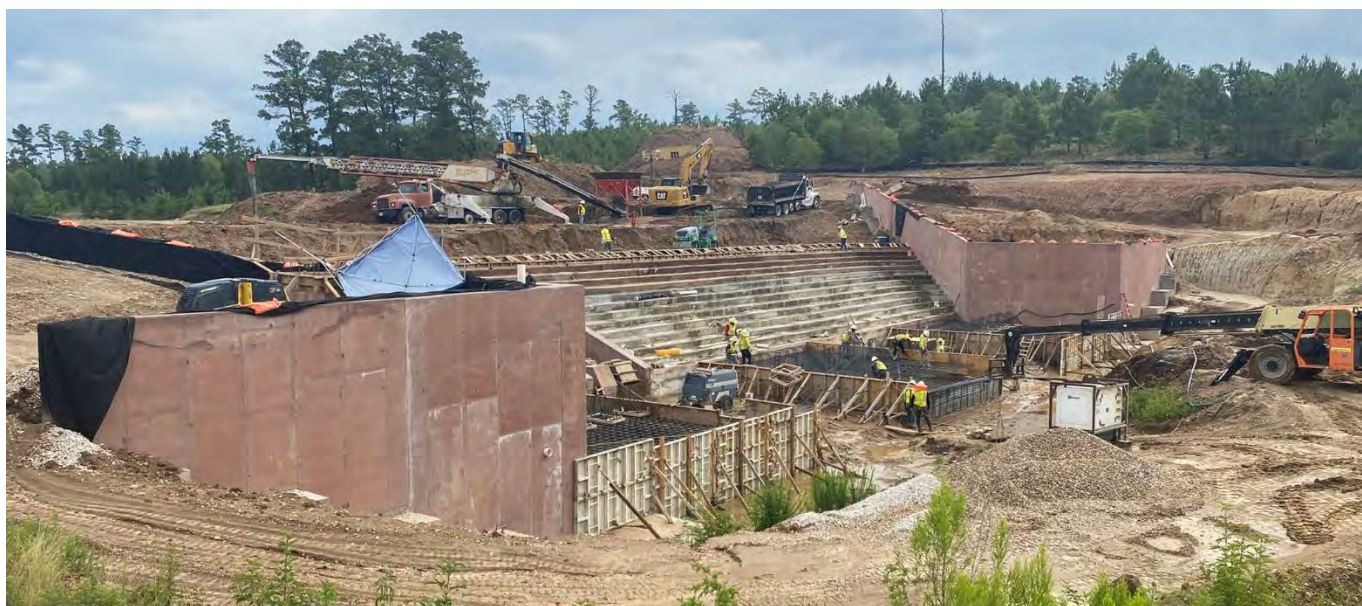
Reconstruction of the Bastrop State Park Dam
