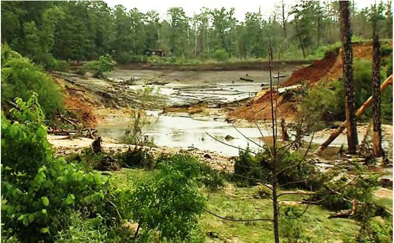
Failure of the Bastrop State Park Dam, which was originally constructed in 1913, during the 2015 Memorial Day flood event. Source. Texas Parks and Wildlife
