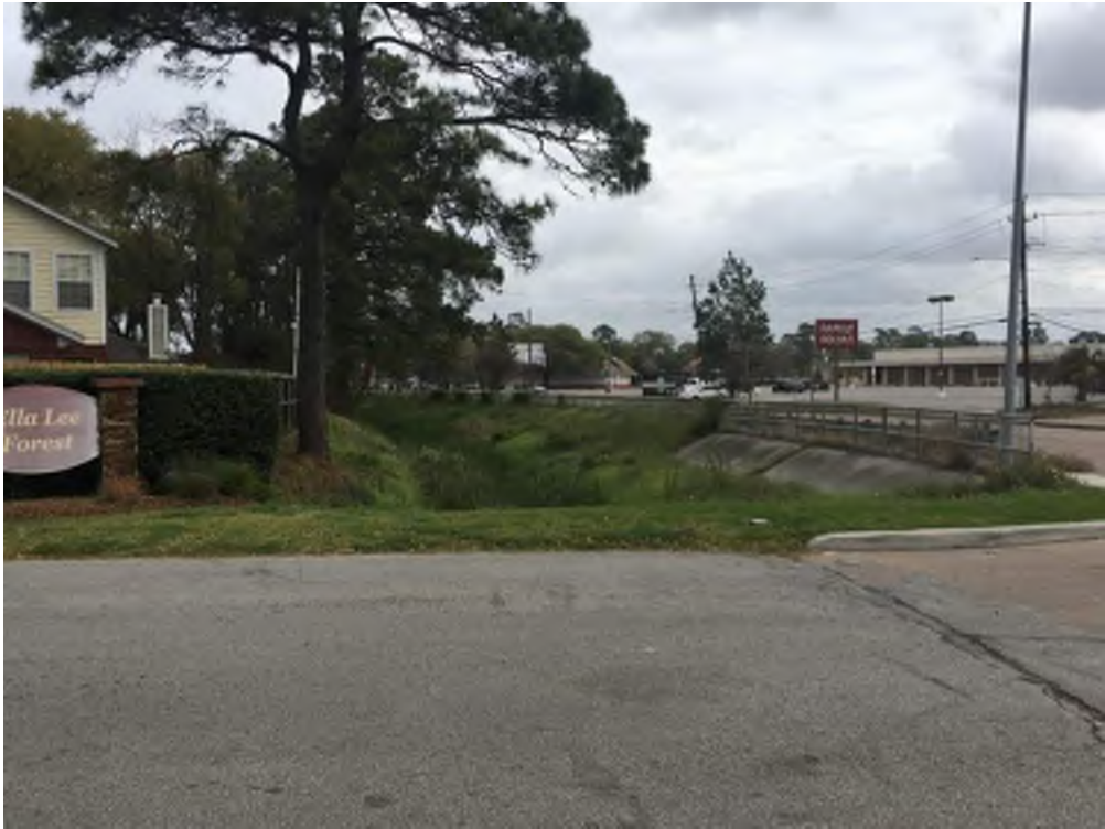
Photo #16: Lehman Road crossing at E116-05-00 looking upstream (PA02)
