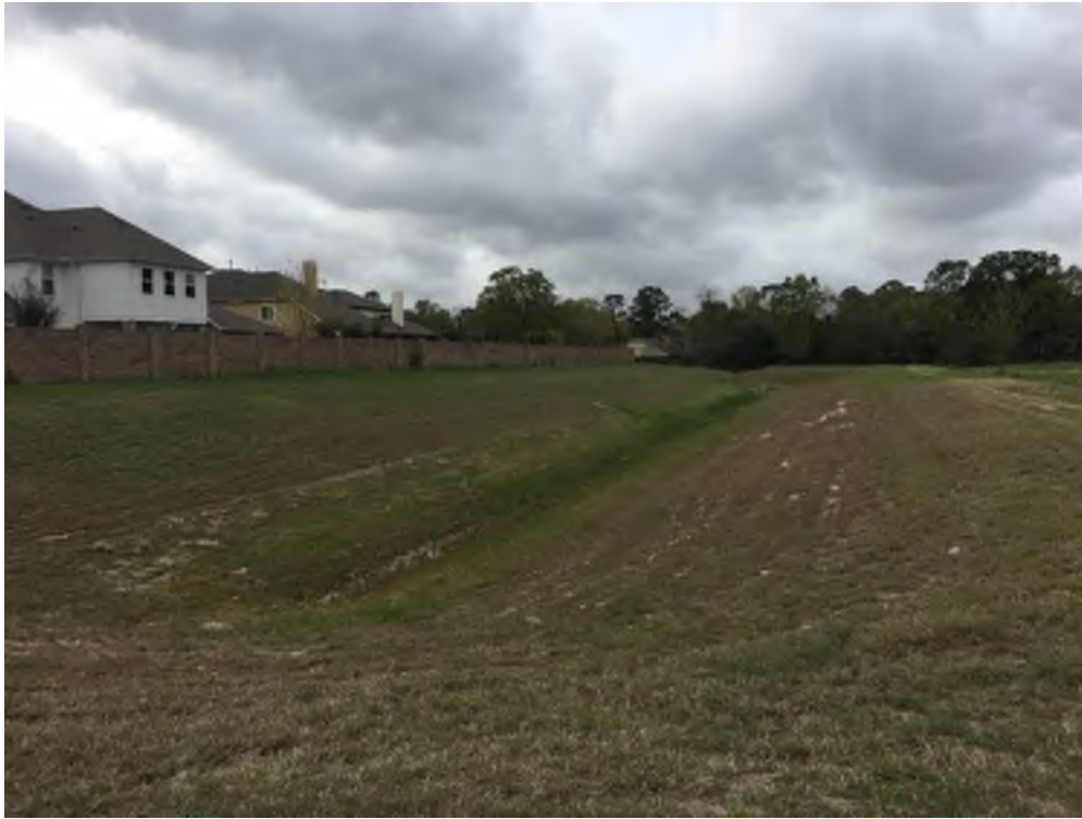
Photo #11: HOA detention basin to the east of HCFCF basin E516-01-00 (PA02)
