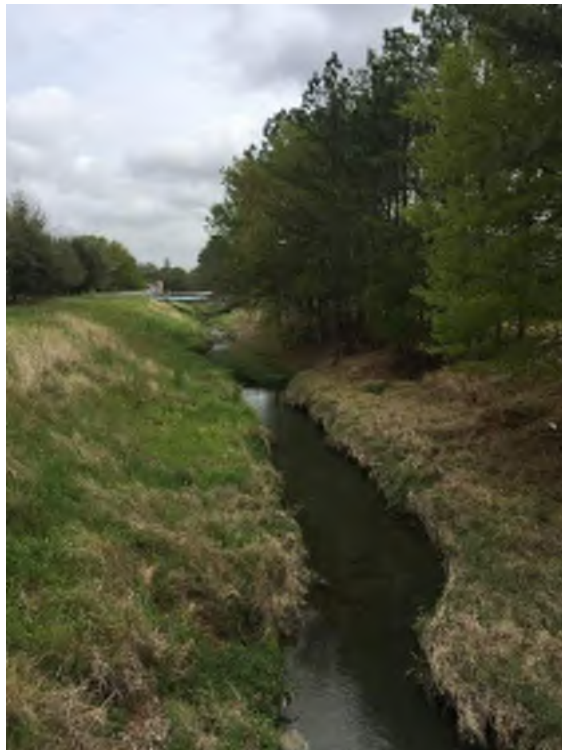
Photo #8: E116-00-00 upstream of Del Norte Street crossing (PA02)
