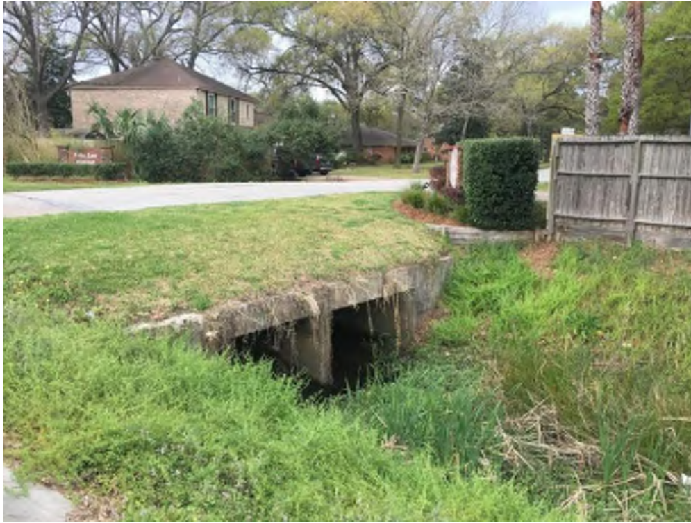
Photo #19: Upstream Face of Lehman Road culvert crossing at E116-05-00 (PA02)
