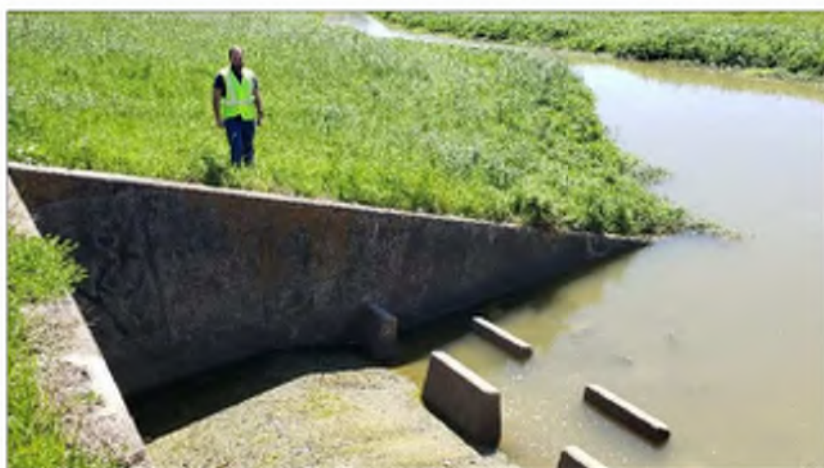
Figure 13. Drop structure at N109-00-00
