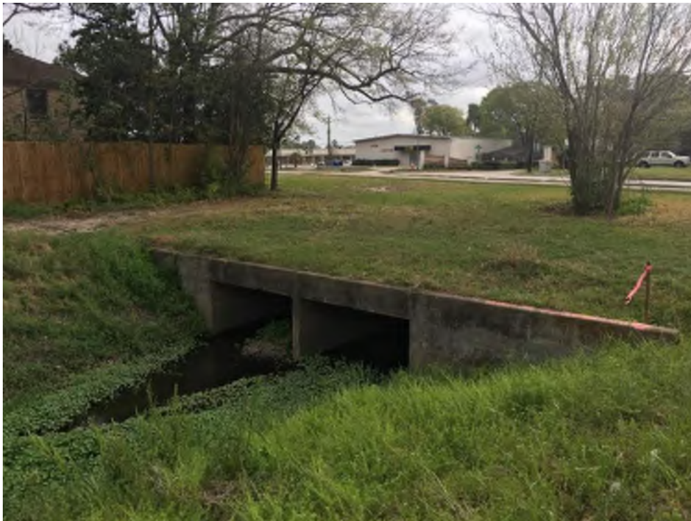
Photo #20: Downstream Face of Lehman Road culvert crossing at E116-05-00 (PA02)
