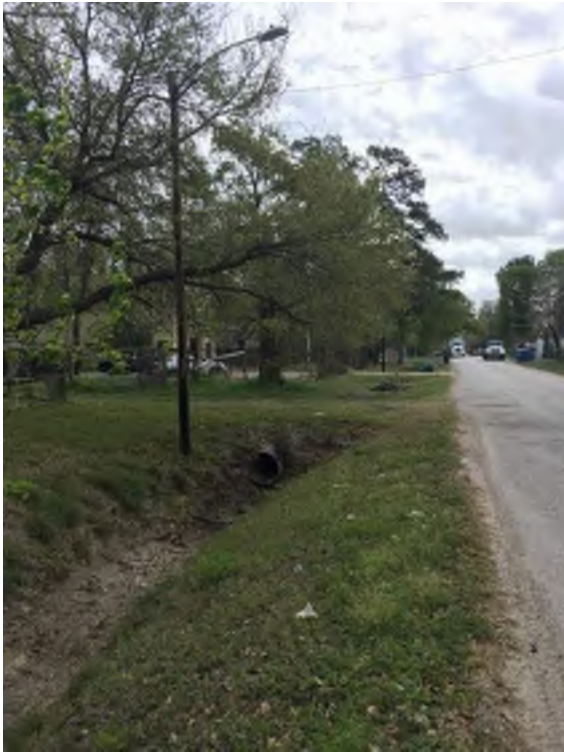
Photo #3: Northern roadside ditch along Paul Quinn Road (PA04)
