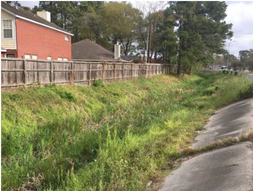
Photo #18: E116-05-00 channel upstream of Lehman Road crossing (PA02)
