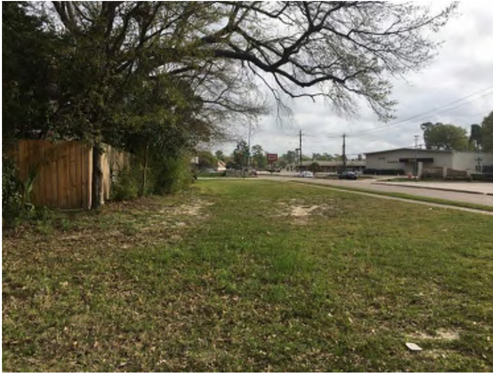
Photo #21: Parkway on top of Lehman Road culverts along E116-05-00 (PA02)
