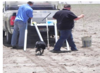
Moisture probe installation
