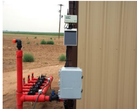
Valve bank with air relief
